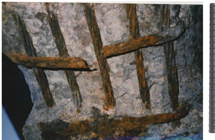
Figure 19: Example of steel reinforcements corroding in conventional concrete. Reproduced from [13]
